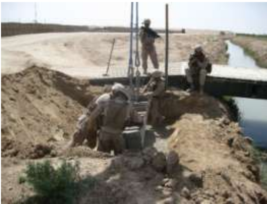
Photo 2. 8th ESB engineers emplacing footers for an ESB designed and built steel and timber non-standard bridge, with the Medium Girder Bridge (MGB) that it will replace in the background.
