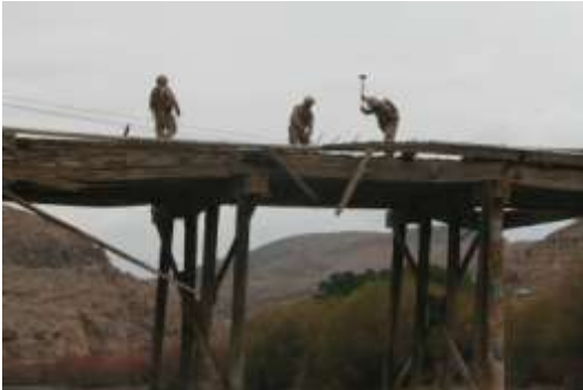
Photo 1: 8th ESB engineers repairing a local non-standard bridge in the Kajaki District.
